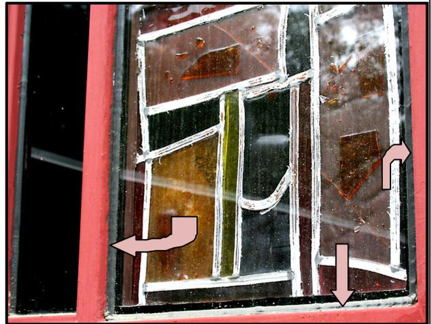
Details showing re-worked window following installation of exterior glass protective coverings over the sanctuary west wall mosaic window. Arrows point to super-sealant applications.
